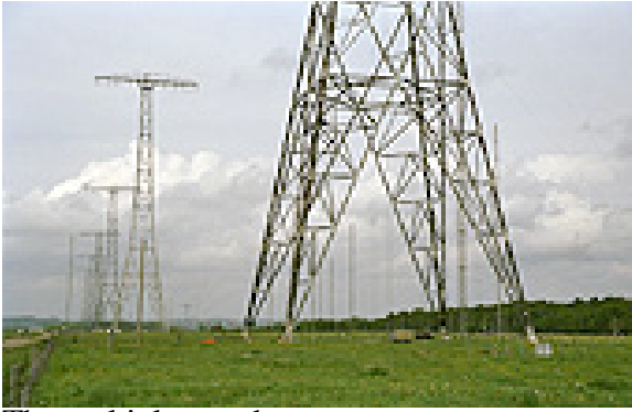
The multiple tuned antenna
